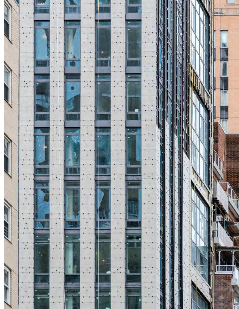
The opaque side of the building features a horizontal layout porcelain rainscreen system
