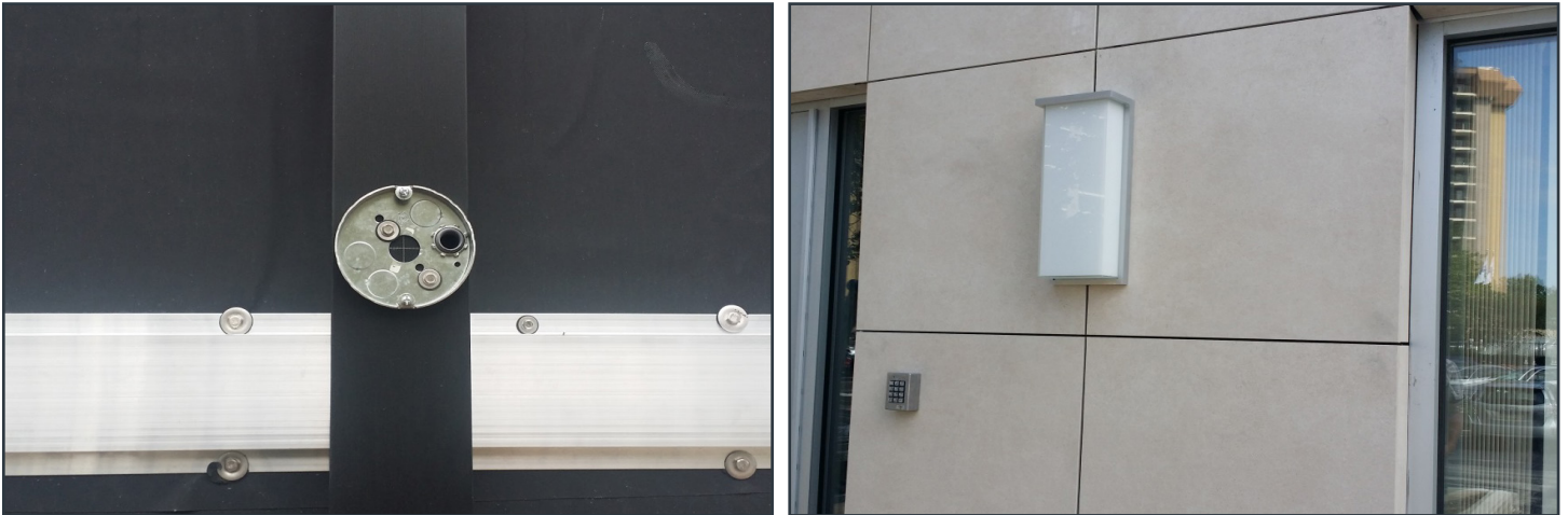
Example of light box installed in a vertical profile, for the installation of a lamp.
