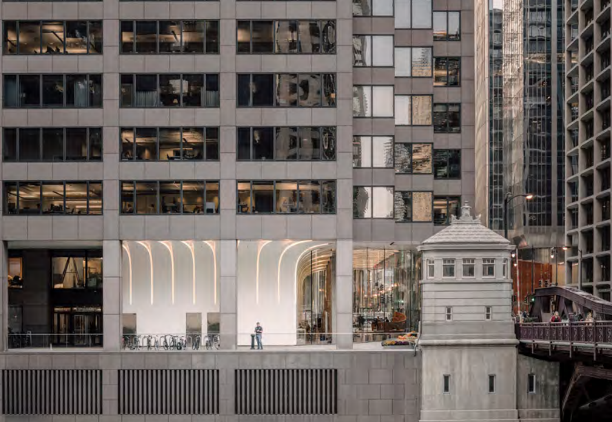
CME Lobby Renovation / Chicago, IL
