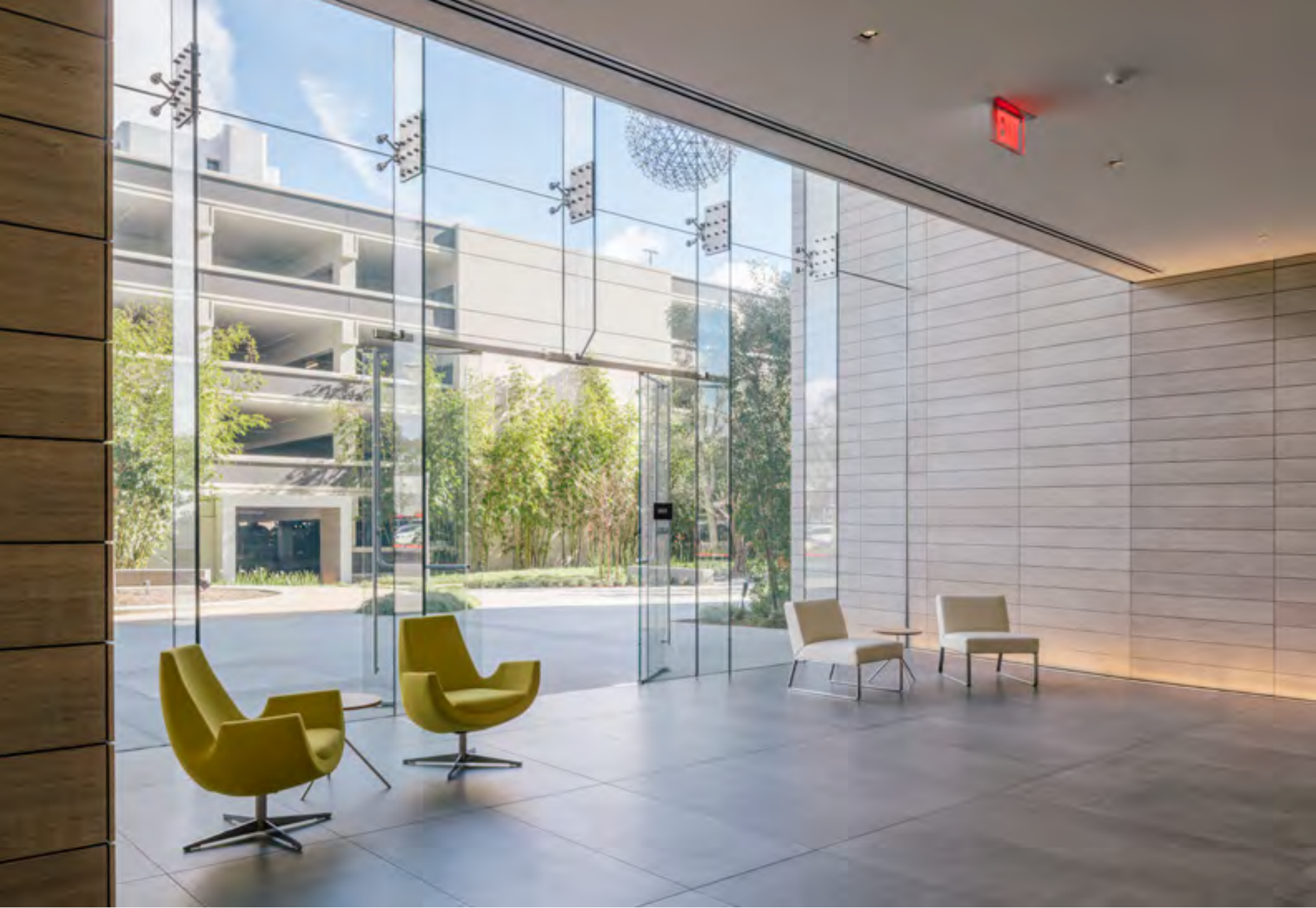
Pacific Center Lobby Renovation / Torrance, CA
