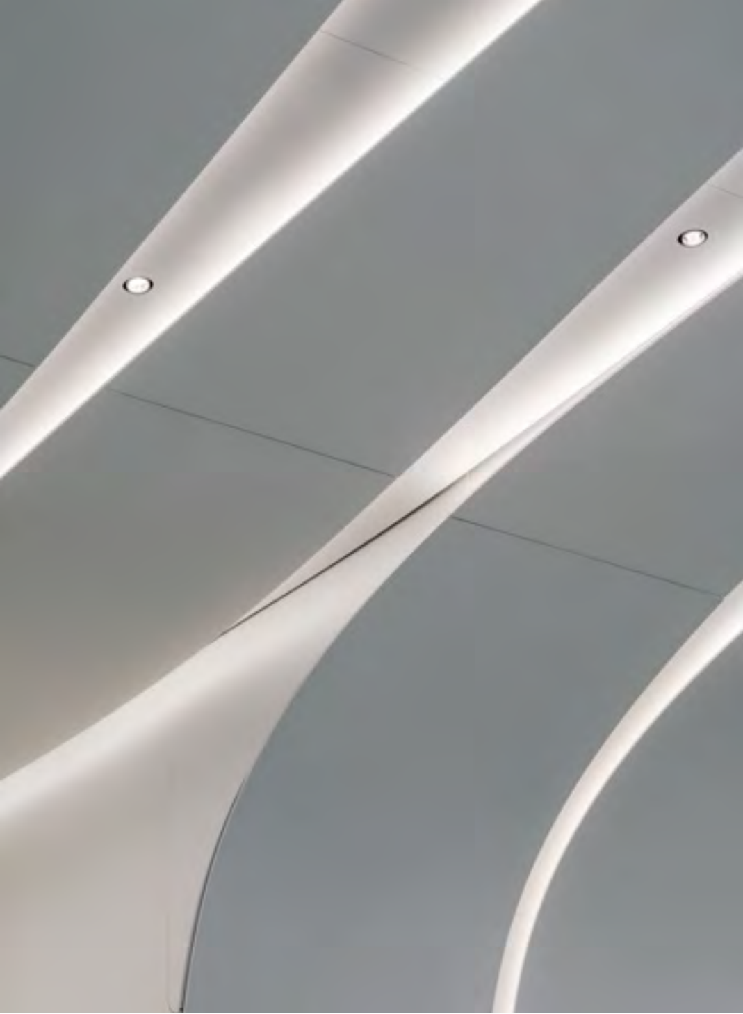
CME Lobby Renovation / Chicago, IL
