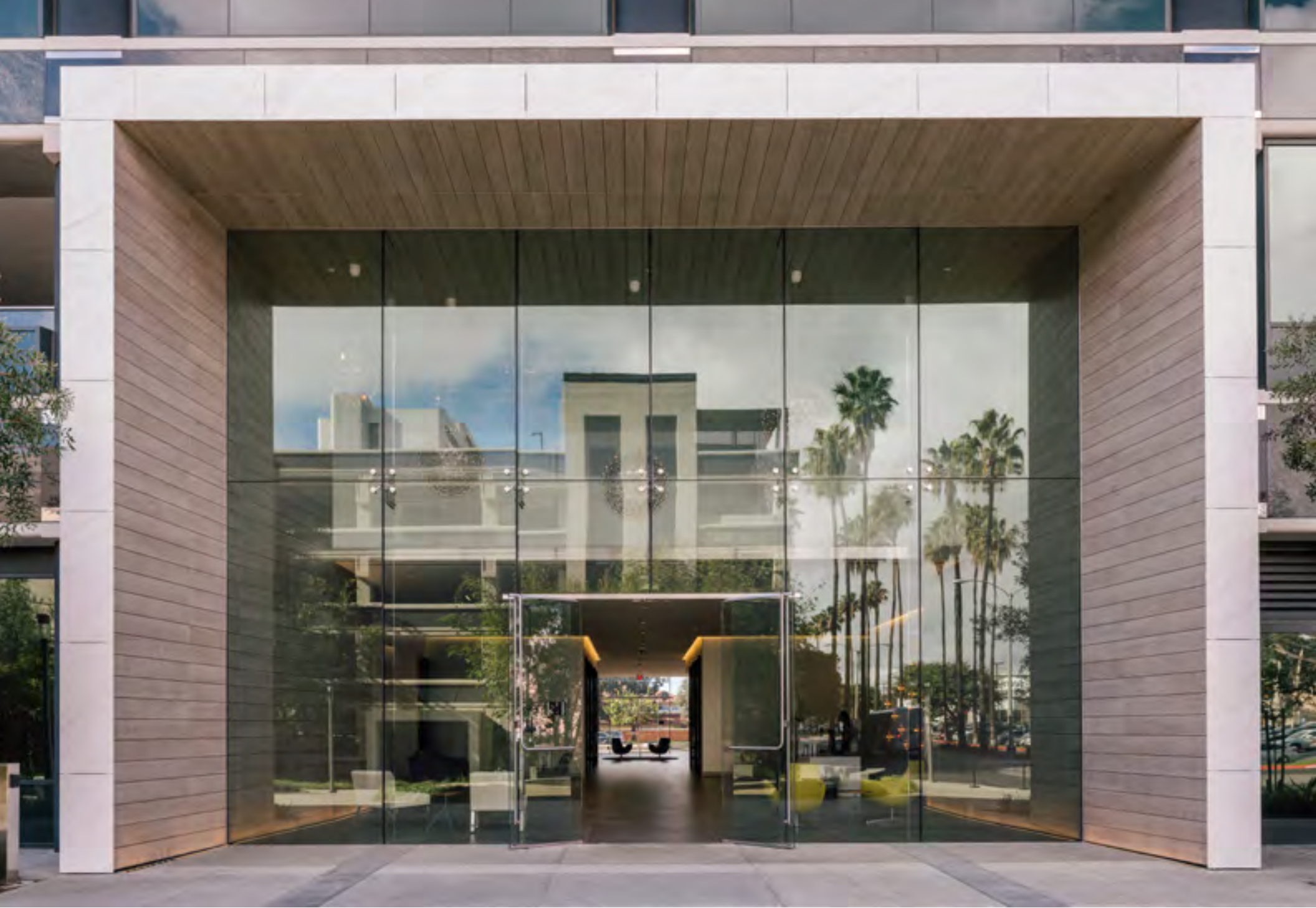
Pacific Center Lobby Renovation / Torrance, CA
