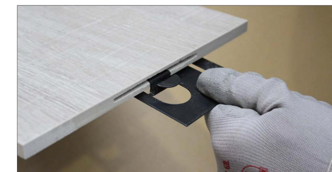
8. Check the panel mechanical resistance is not compromised and that the clips fit in the kerf.
